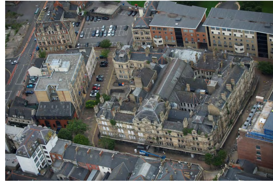
AERIAL PHOTOGRAPH FROM EAST
